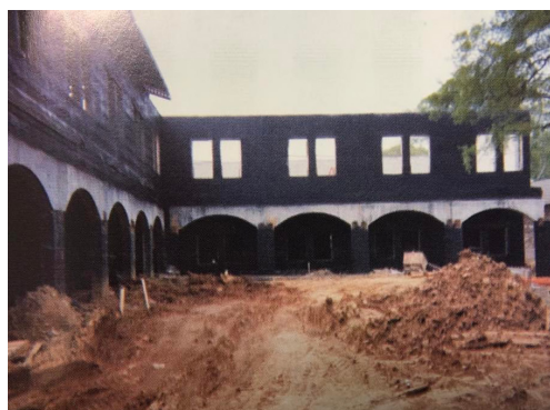
SCGSAH residential campus courtyard under construction
